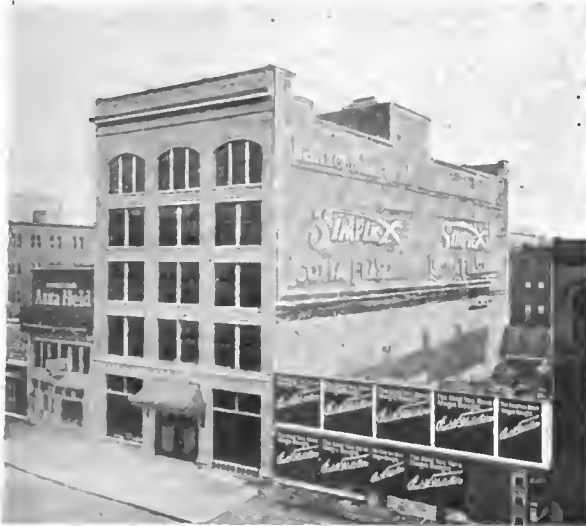
BROADWAY ENTRANCE TO BUILDING.
